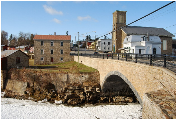
Keystone Arch Bridge- Keeseville
